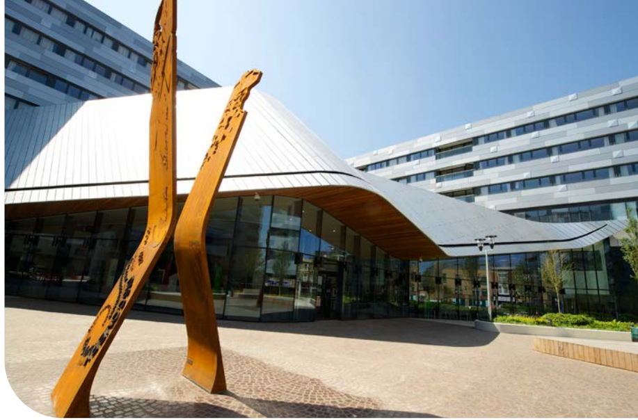
The London Centre's entrance
